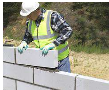
(Fig.111 Thin joint Masonry)
