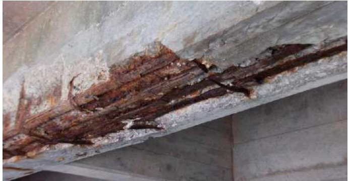
(Fig.35 Corrosion of Beam)
