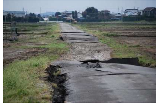
(Fig.32 Soil Liquefaction)
