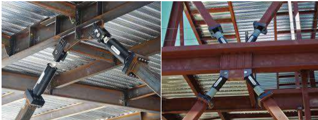
(Fig.100 Seismic Dampers)
